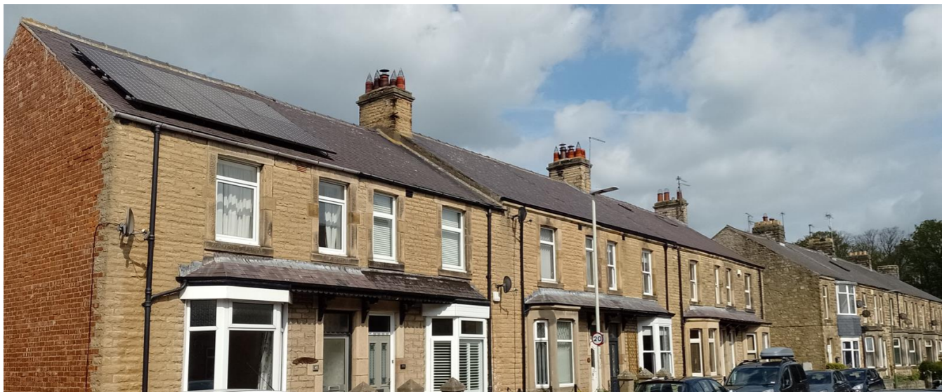
Solar panels on terraced street
